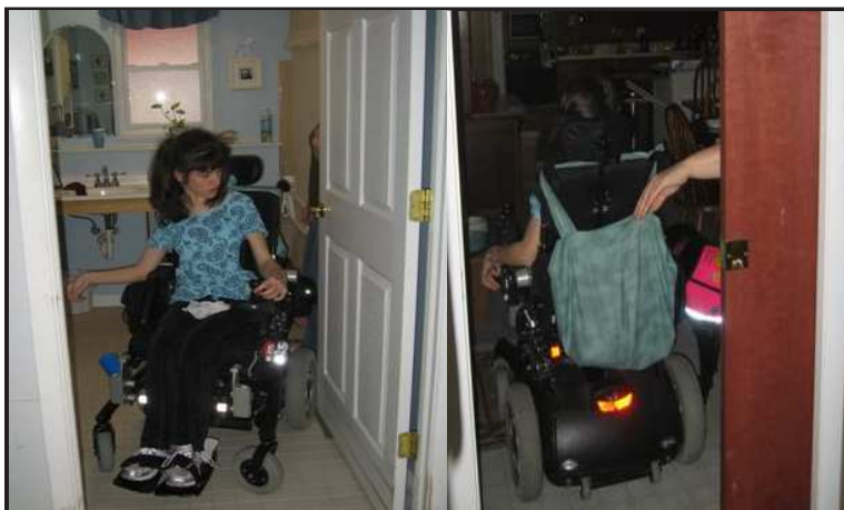
Allison maneuvers easily in the accessible bathroom with its smooth, flush threshold, and enjoys the wheelchair-friendly sink configuration. The former vanity sink was located along the left wall and was removed. Right, a 'pocket door' provides privacy for the therapy room (see photo, p. 6) without getting in the way. Princess, wearing the hot pink reflector jacket, stands ready to assist Allison.
